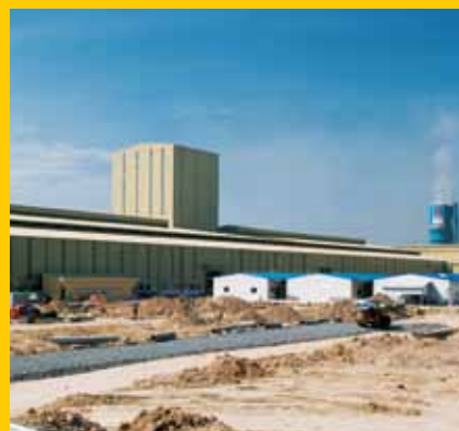
The construction site of Hoa Sen – Phu My Steel Sheet Plant
